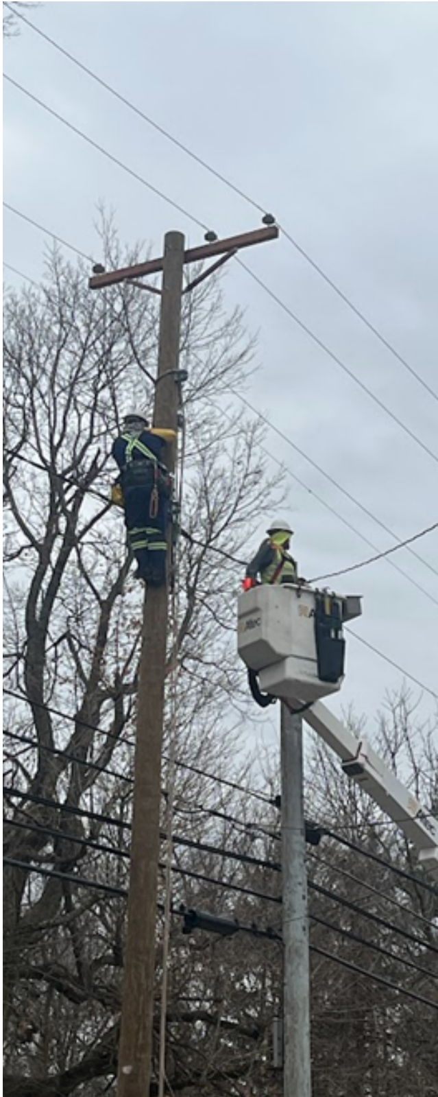
Recent electric and metering projects.
